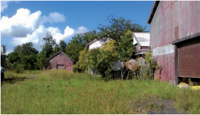
Photographic Plate 20: (Viewing Location 20) View south on alignment of former Creamery Station spur line
