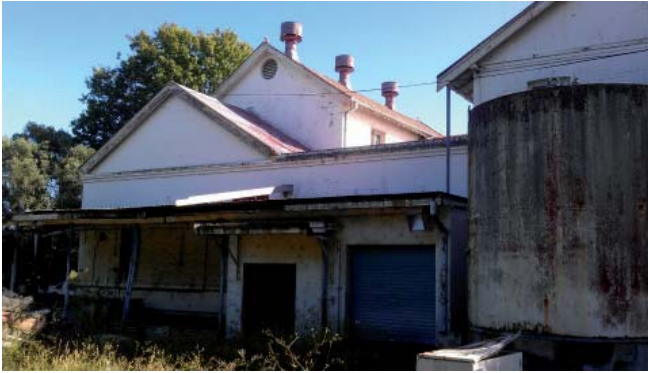
Photographic Plate 21: (Viewing Location 21) Handling area of Creamery Building
